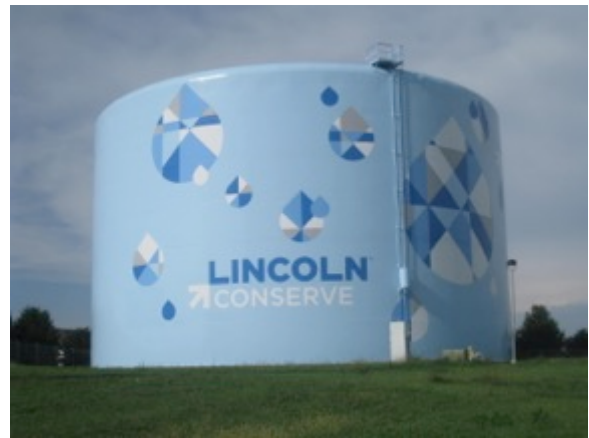
One of Lincoln’s water reservoirs at 56 th and Pine Lake Rd.
