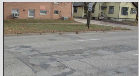
Temporary patching of the failed asphalt surface
