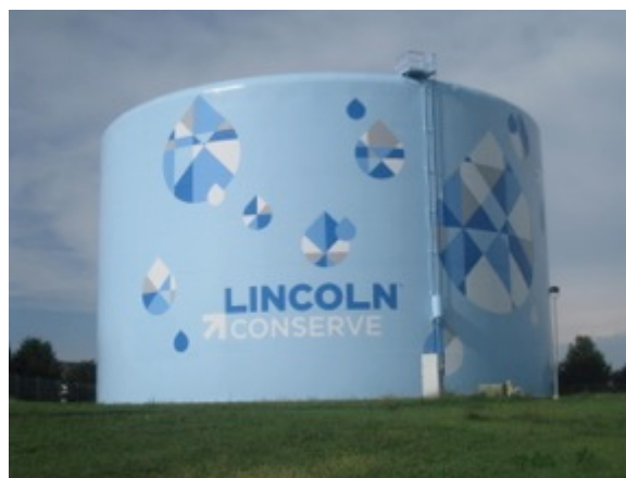
One of Lincoln’s water reservoirs at 56 th and Pine Lake Rd.
