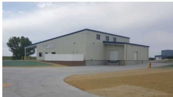
The new Hazardous Materials Collection Center at the N. 48 th Street Solid Waste Facility.
