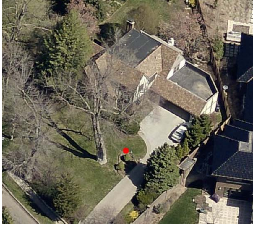
Aerial from south of 2340 Woodsdale, 2013
