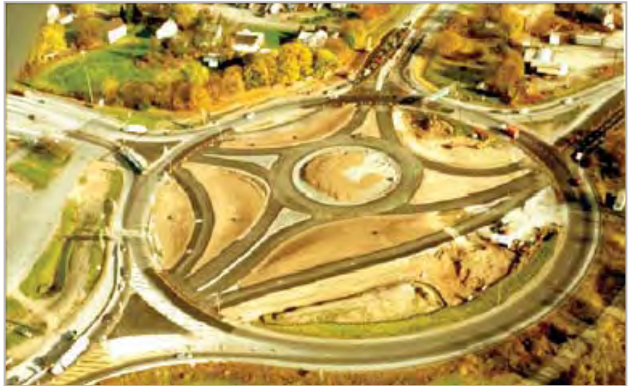
..... Note the new modern roundabout being built inside of an old traffic rotary in the picture above.
