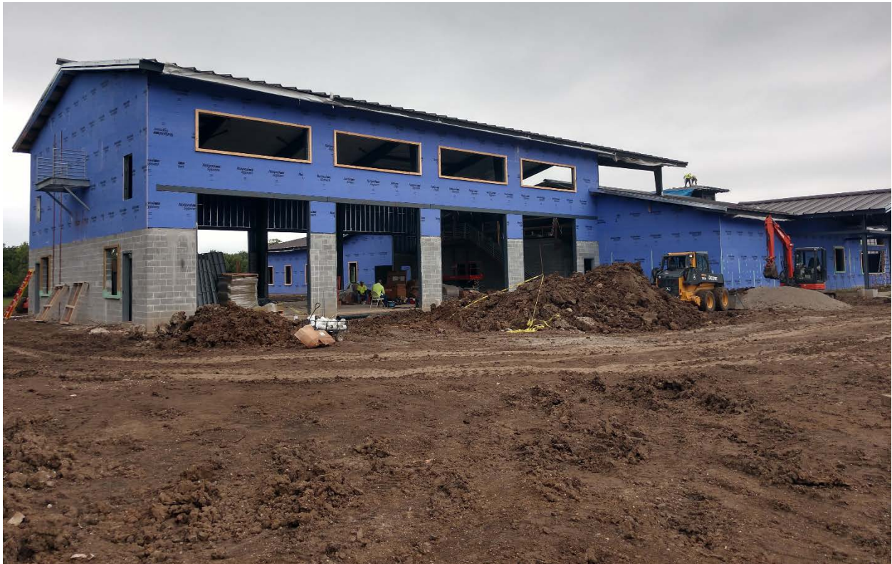
*Construction progress on the new LF&R Station 15 as of 8/30/2018
