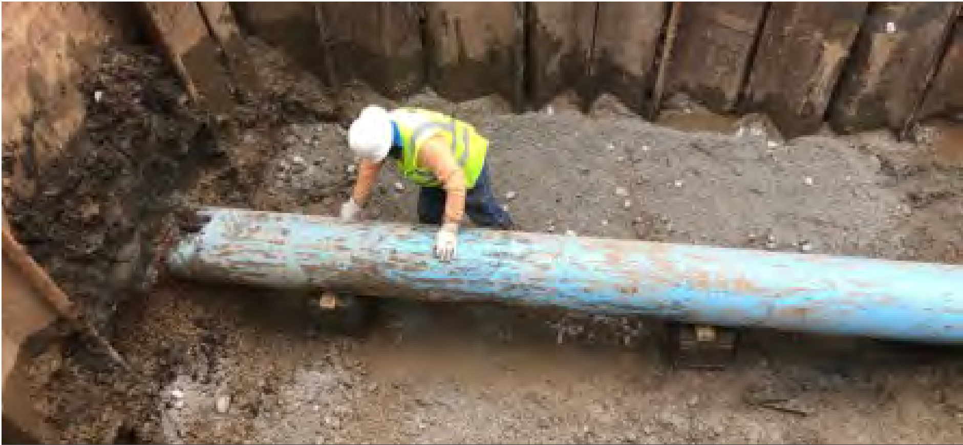
Water main work
