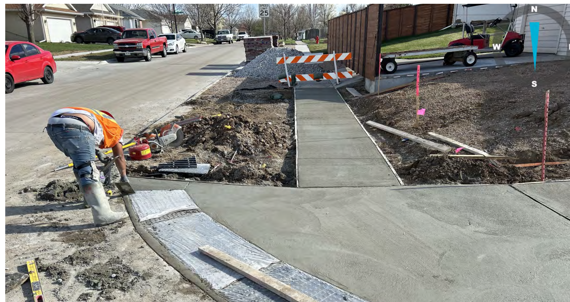
Bikeway & ADA Ramp Construction
