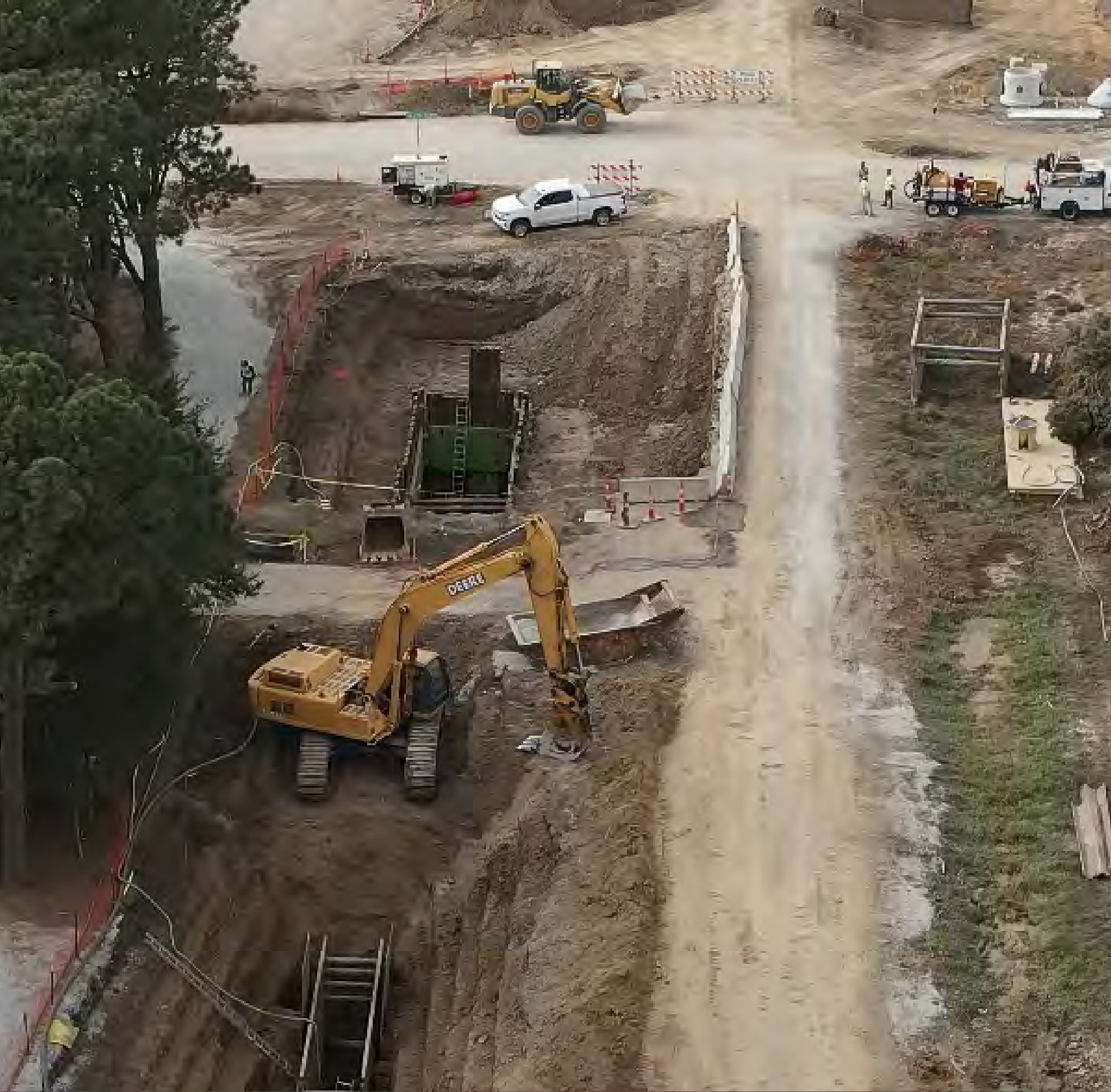
Sanitary sewer installation
