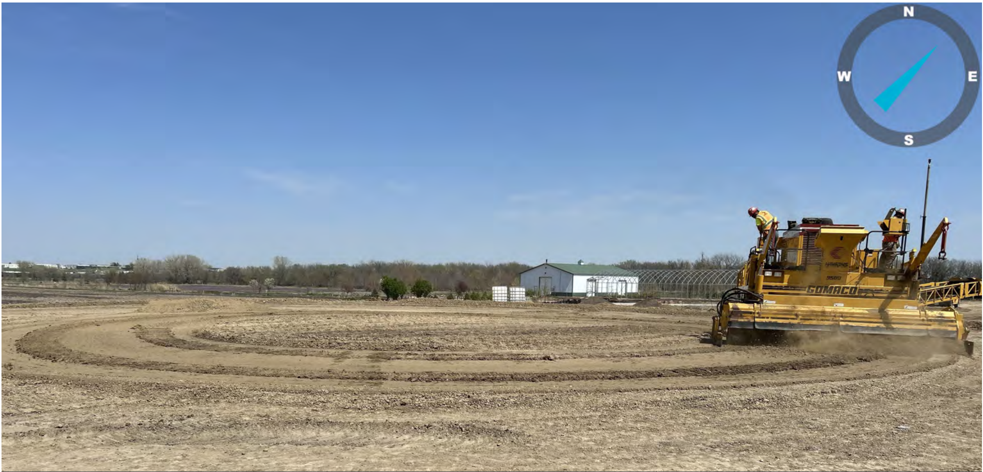
SW 31st St (Paving) Prepping Subgrade For New Roundabout
