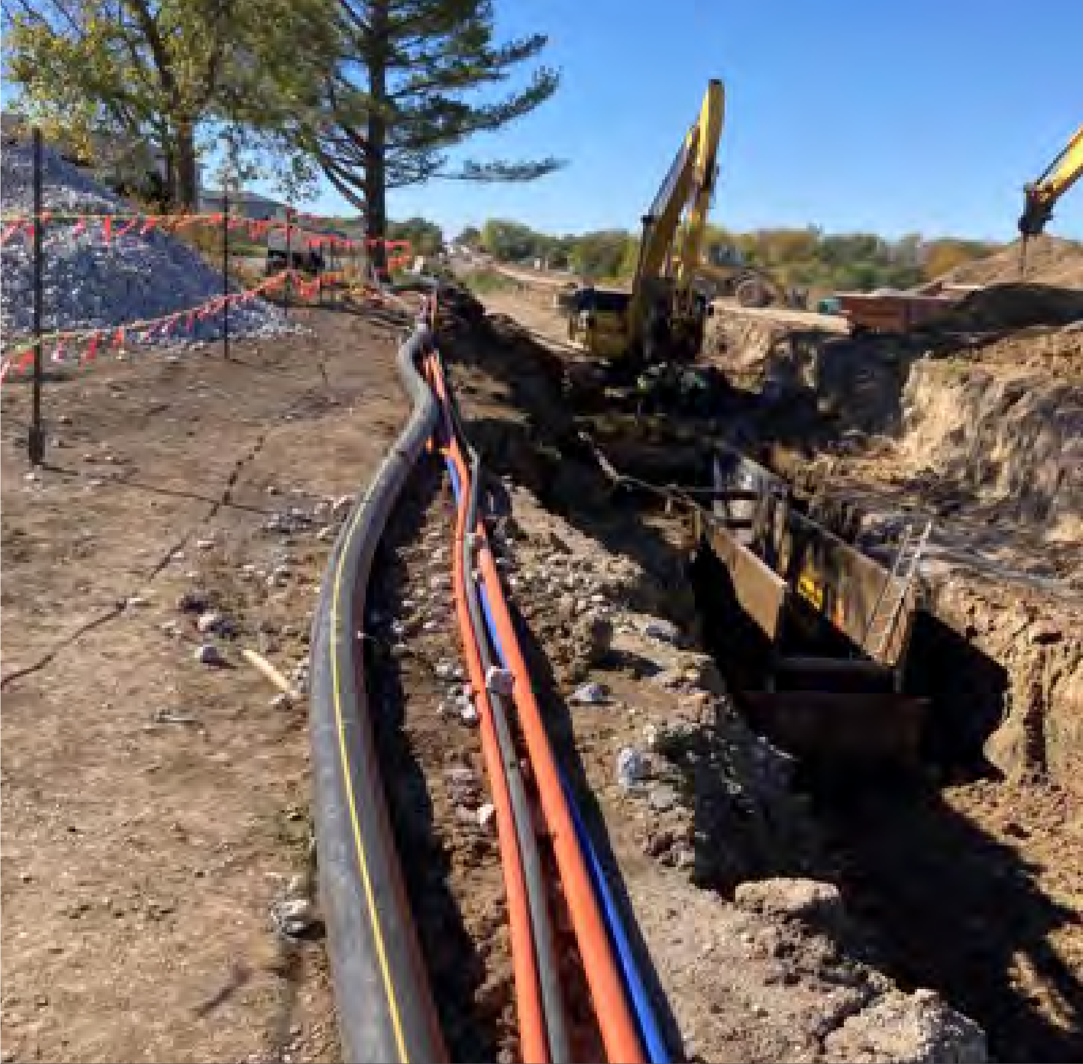
Additional utilities work
