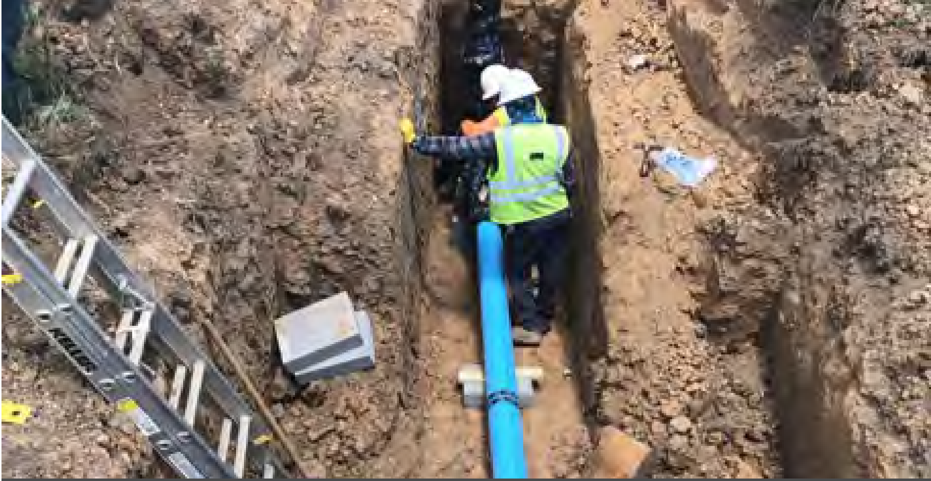
Water main work
