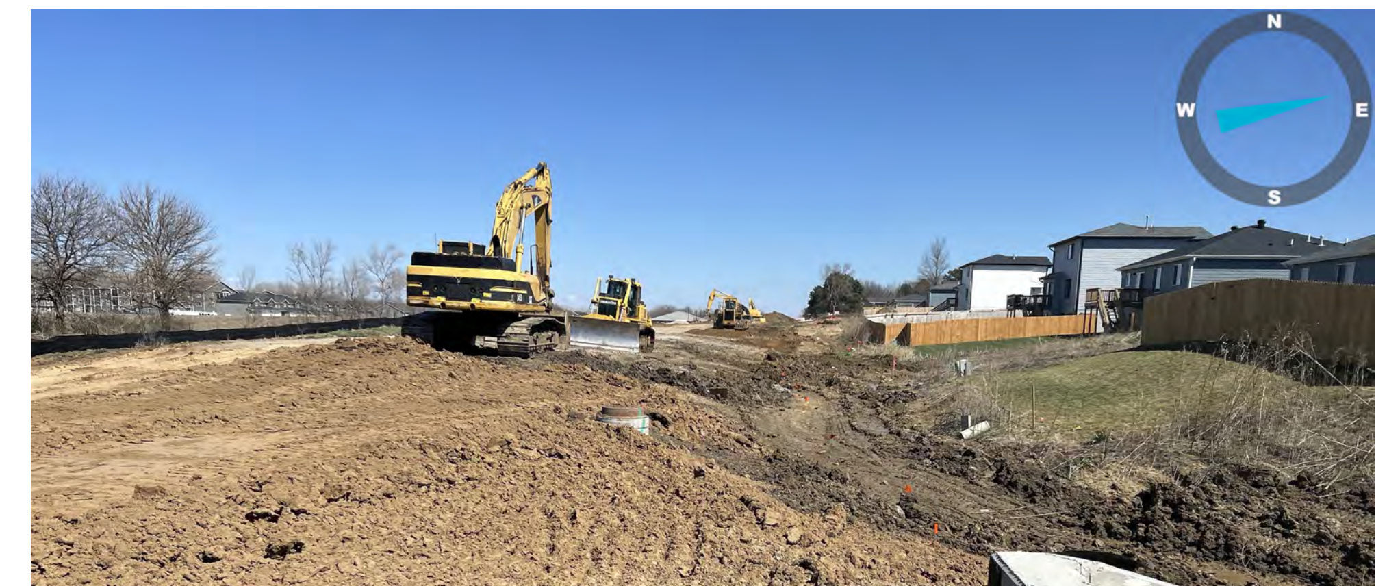
Dirtwork & Widening of West A St. Occurring
