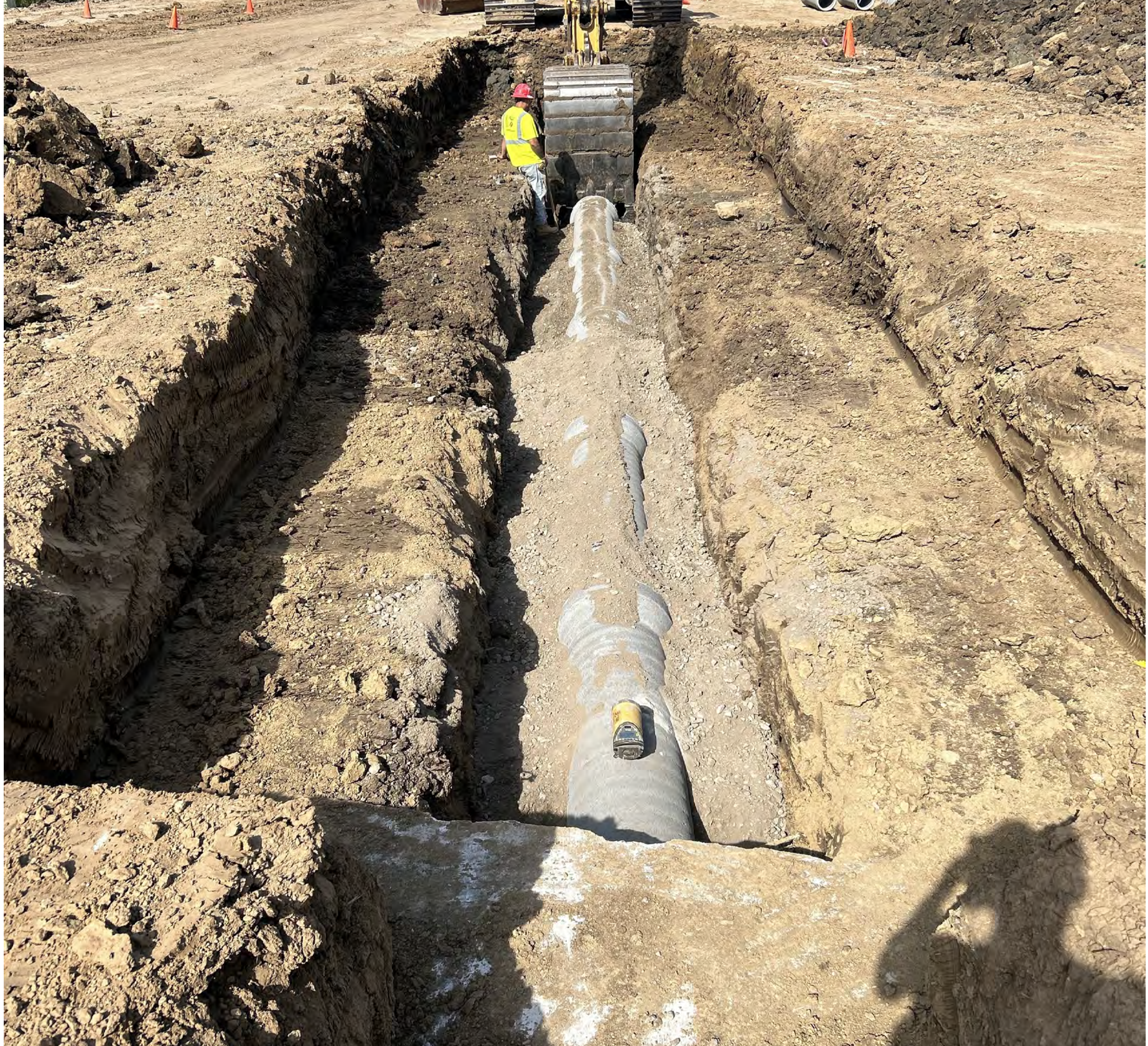
New Storm Sewer Work Between SW 31st to SW 27th
