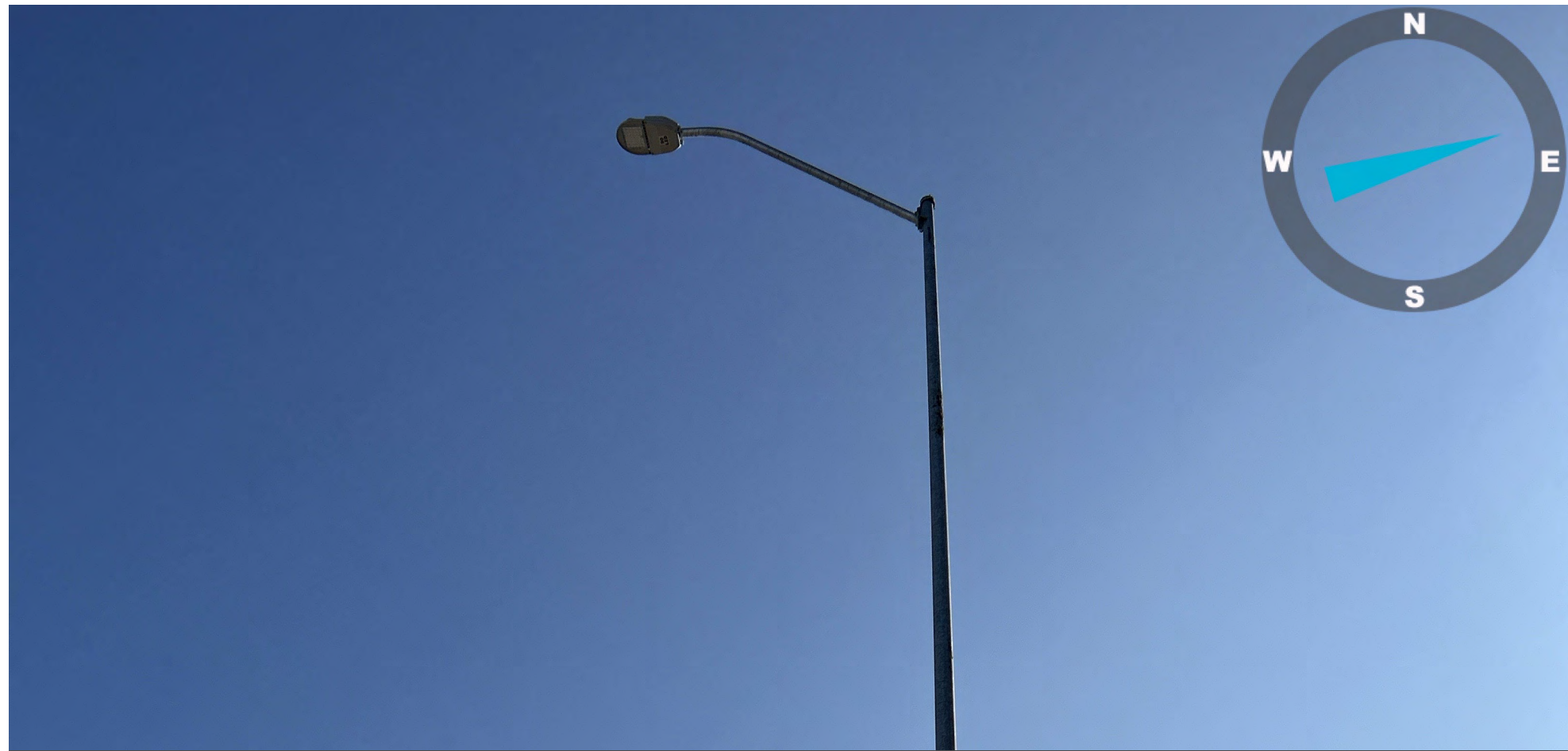
Street Lighting, Signage, Striping Work From City Limits to Timber Ridge
