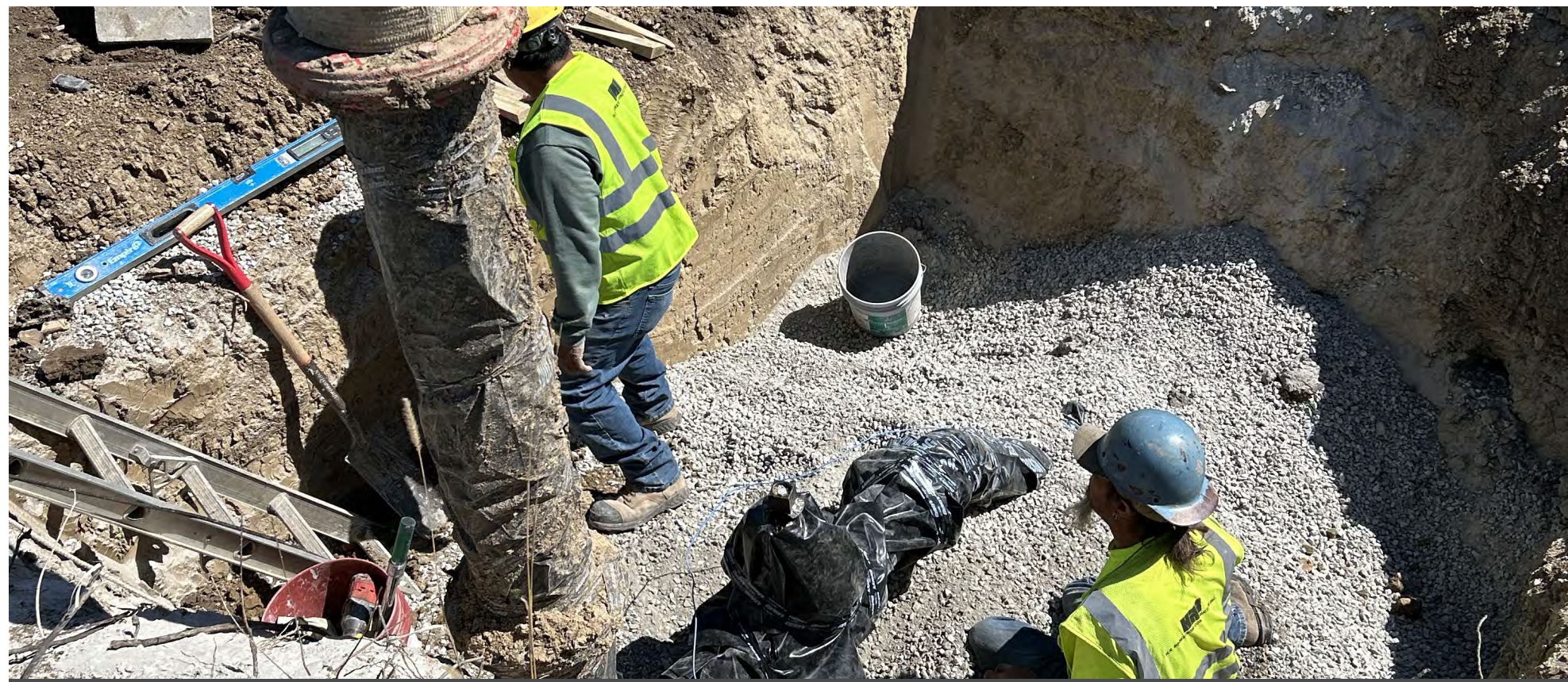
Water Main Work Complete Between SW 36th to SW 31st
