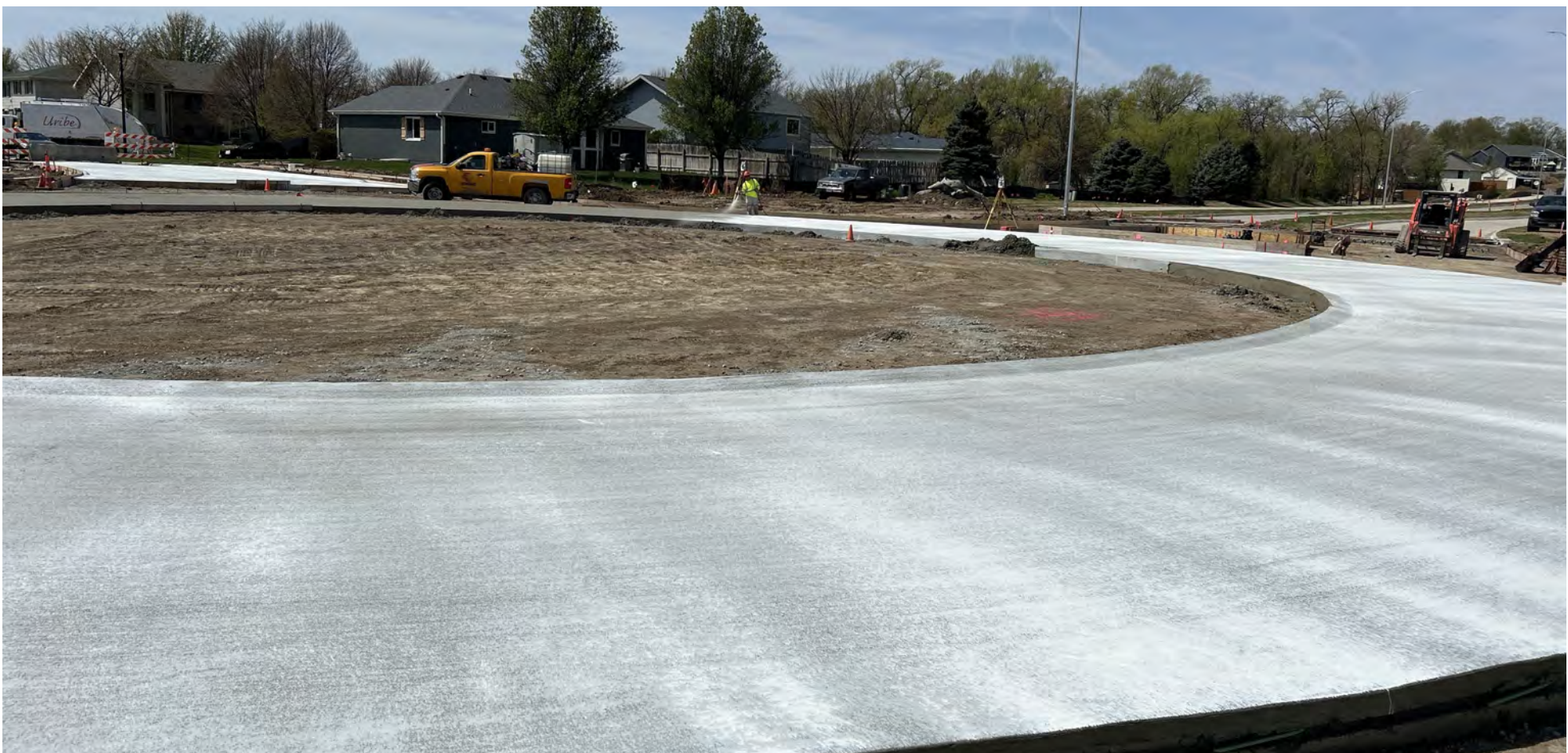
SW 31st St (Paving) Roundabout
