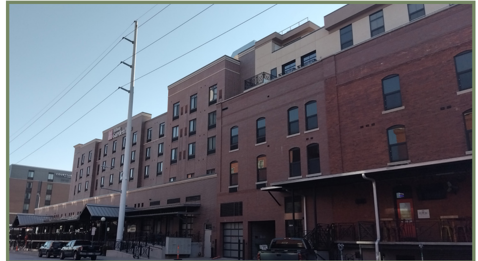
The new Hilton Garden Inn located on 8th Street in the Haymarket Historic District is compatible with the district but can clearly be seen as a modern building. The dock height is continued along the new facade replicating the design of the Henkle and Joyce Building. The brick is distinguished with a new color and the offsets on the facade reduce the overall massing.
