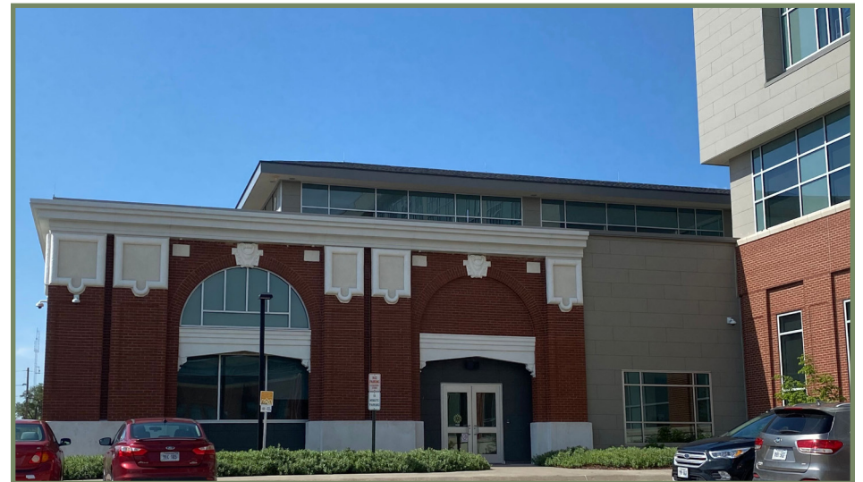
The additions to the Industrial Arts Building is an approach that deviates from the historic character by stepping back from the main facade with a neutral colored palette.
