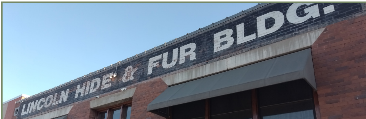
Maintenance of the Lincoln Hide and Fur Building signage shown above.
