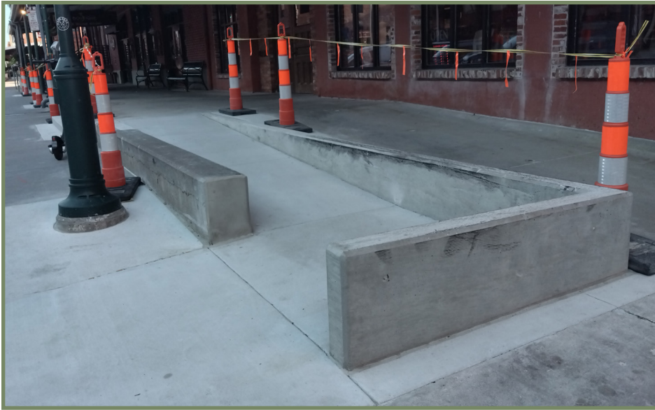
The above ramp was installed to provide ADA access to the businesses in the historic district. The low profile of the ramp walls avoids obscuring the facade of the adjacent historic buildings.
