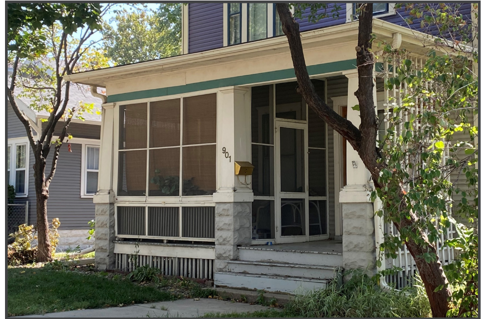
The partially enclosed porch above retains the original railings, columns, and visibility to the front facade.
