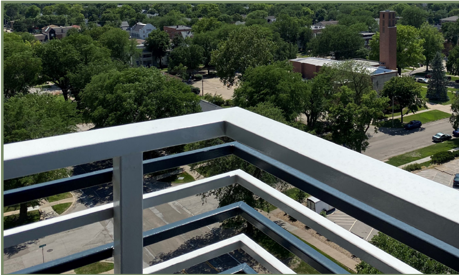
To meet code requirements on guard rail spacing, the Sky Park Manor project added the additional horizontal black rails which fade into the background, allowing the original aluminum rails to stand out.
