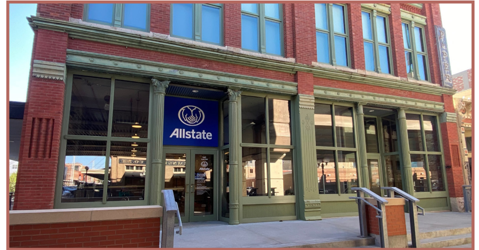
The 1884 Schwarz Paper Building at 747 O Street features a cast iron storefront with engaged Corinthian colonettes, central pier, rosettes and terra-cotta capitals.
