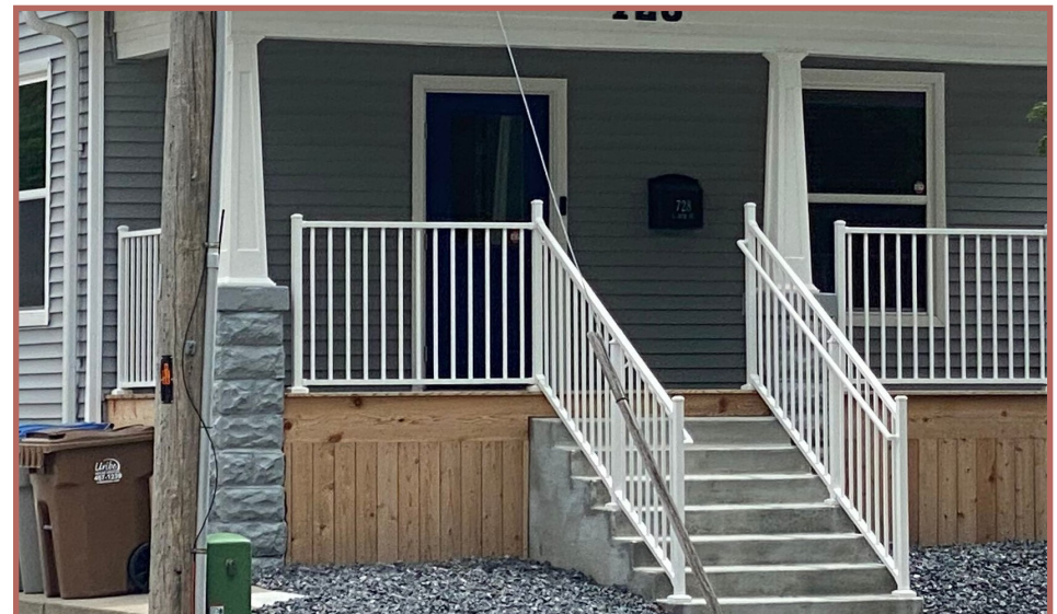
The porch skirting and railings above are not an appropriate treatment for a historic building. The square columns that replaced originally rounded columns illustrate the panel design with base and cap concept, however the tapered design is not true to the prairie box style of the home.
