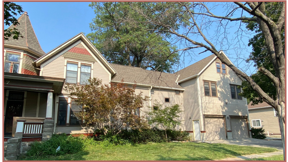
The two story link with three story garage addition competes with the original home in overall scale and massing, however the neutral color palate and matching roof pitch with step back in the link portion are in alignment with the historic home.
