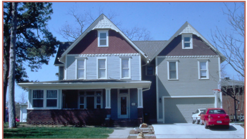
The addition to this home for the garage has similar results as above, also with the problem of a modern garage competing with the main porch and entrance to the home given the close proximity.
