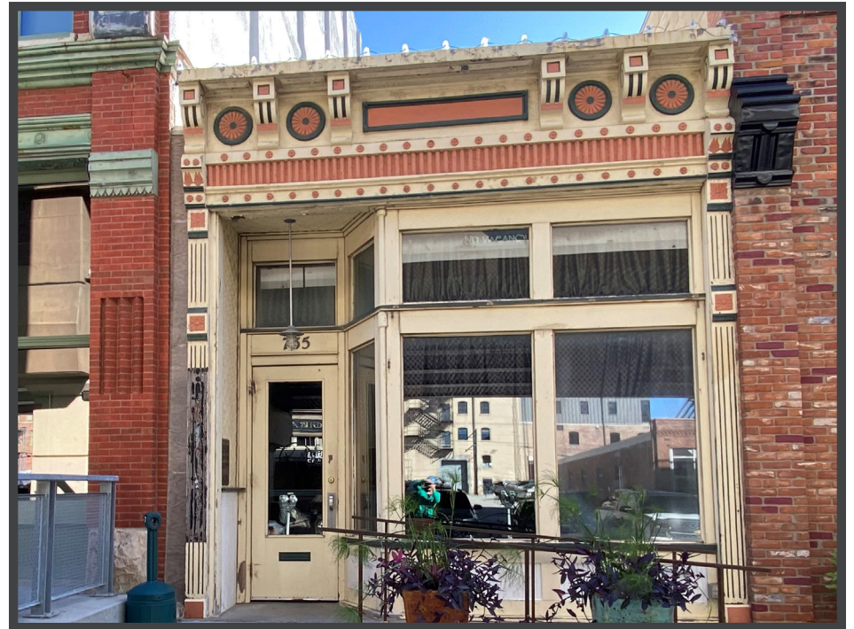
The Occidental Saloon at 735 O Street appears to also be cast iron but is instead the Victorian storefront is carved out of wood.
