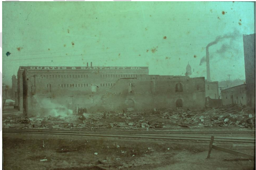
Figure 6: Fire at the Curtis and Bartlett Building
