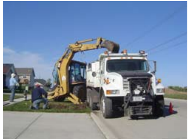
Sanitary Sewer Maintenance
