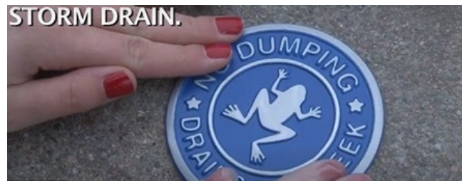
Keep Lincoln Lancaster County Beautiful works with volunteer groups to install Storm Drain Markers on area inlets
