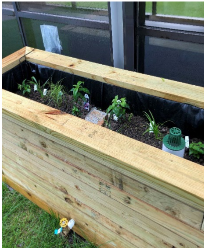
Planter at Municipal Service Center (MSC)
